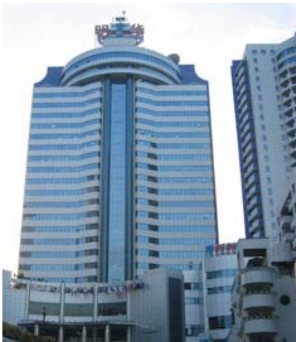
MING WAH International Conference Centre, Shenzhen, China
